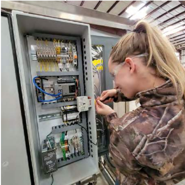
Megan, Spire Electrical Assembler tightens up her work on a PRIMUS Sterilizer by Spire Integrated Solutions.
