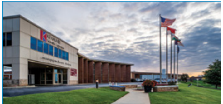
Kewaunee Headquarters & USA Manufacturing Facilities: Statesville, North Carolina
